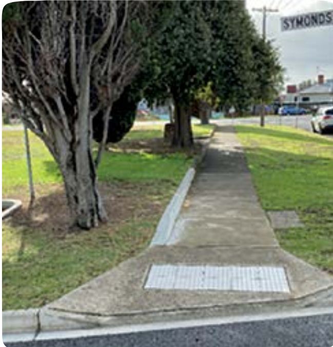
DDA compliant kerb ramp
