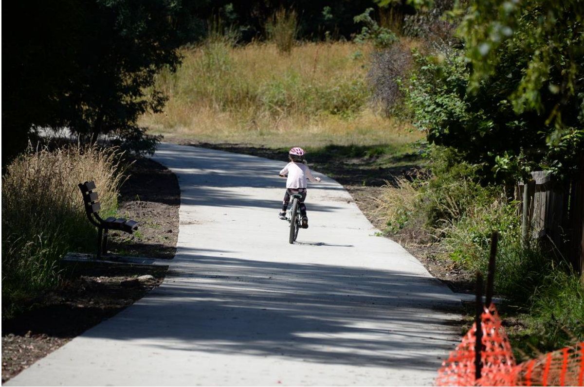
Photo: new Whitewater Creek path allowing a safe route between Huntingfield and Kingston.
