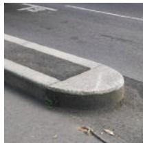
Concrete separator island
