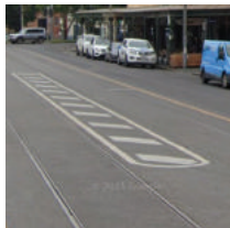
Road narrowing/painted island
