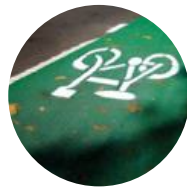
GREEN SURFACE PAVEMENT TREATMENT
