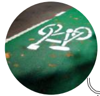
GREEN SURFACE PAVEMENT TREATMENT
