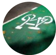
GREEN SURFACE PAVEMENT TREATMENT
